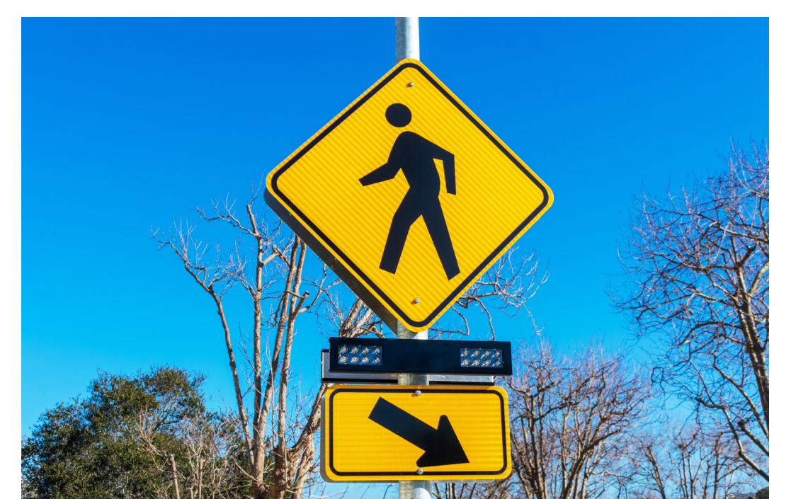
Rectangular Rapid Flashing Beacon (RRFB)
