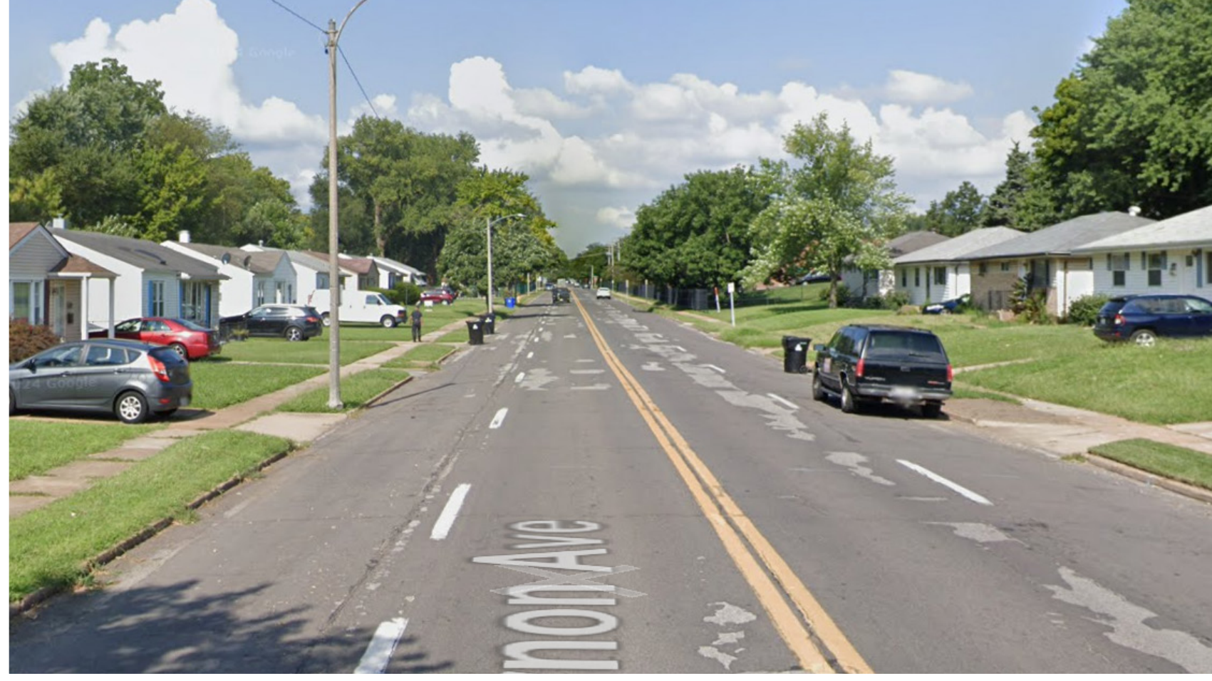
EXISTING CONDITIONS Looking West from Ferguson Ave. & Vernon Ave.
