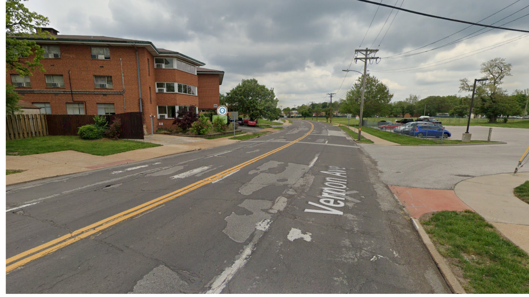
EXISTING CONDITIONS Looking west from Vernon Ave. & Westgate Ave.
