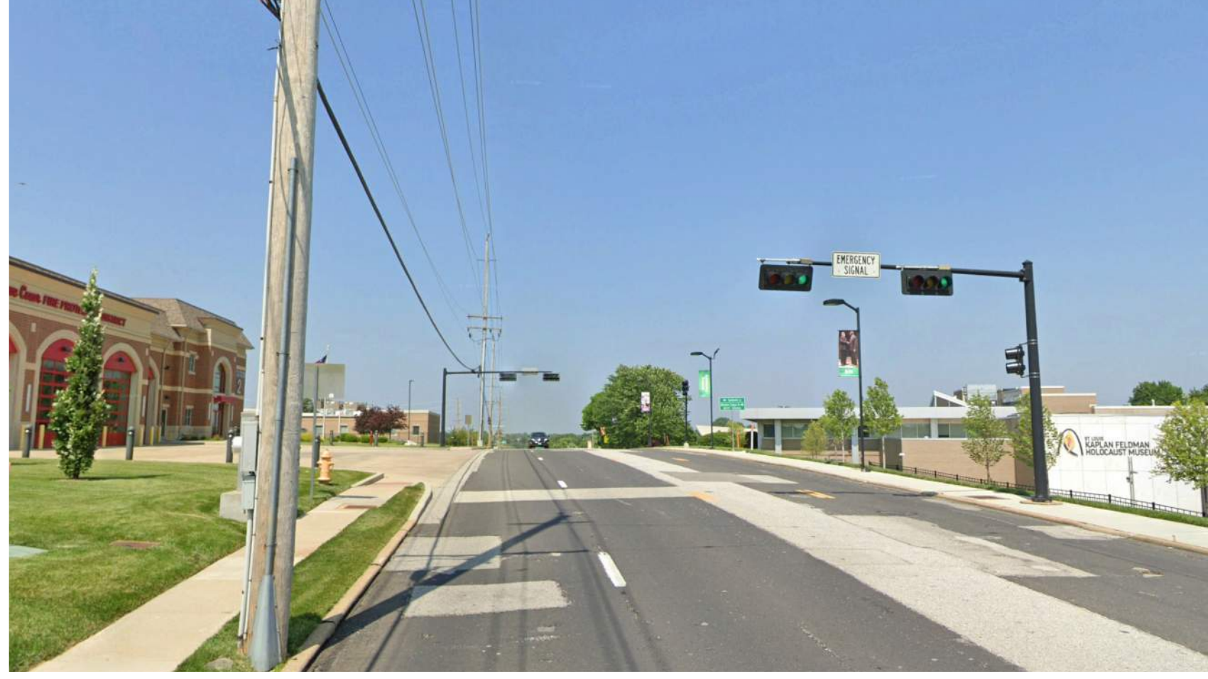
EXISTING CONDITIONS Looking West between HWY 67 & Guelbreth Lane
