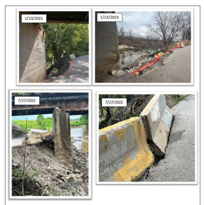
Complicating the project, the geomorphological processes are impacted by Maline Creek's concrete-lined channel, rock bank, a man-made plunge pool downstream of the railroad bridge, and the proximity and frequency of the Mississippi River's backwater effect that need to be carefully considered. The City of St. Louis' Streets department barricaded the damaged area, and we will continue to monitor the damage and restrict Trail Use if conditions worsen.
