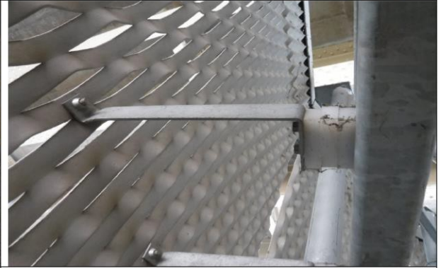
Photo 40 : Typical Connection at Fence – Light Structure
