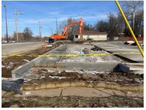
Construction of the new parking lot north of Trojan Park is moving along. The contractors took advantage of late season warm weather to continue excavations and sub-base preparations before the ground temperatures became too cold to move earth. Concrete was poured while possible and the layout for the parking lot, including its permeable paving parking stalls, is now legible to passersby. In the background, the design team is working with the fabricators of the
