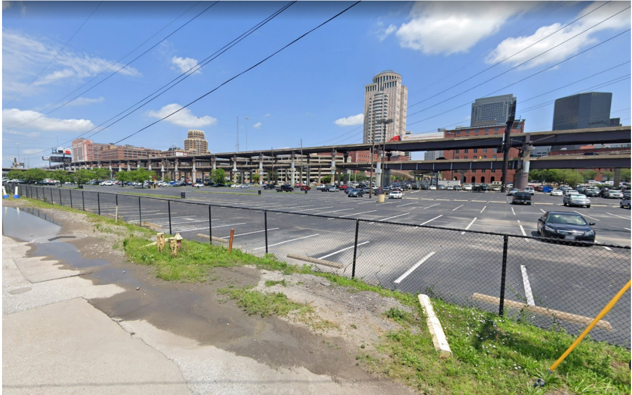
Existing site conditions - Fence and missing curb stops along Cerre
