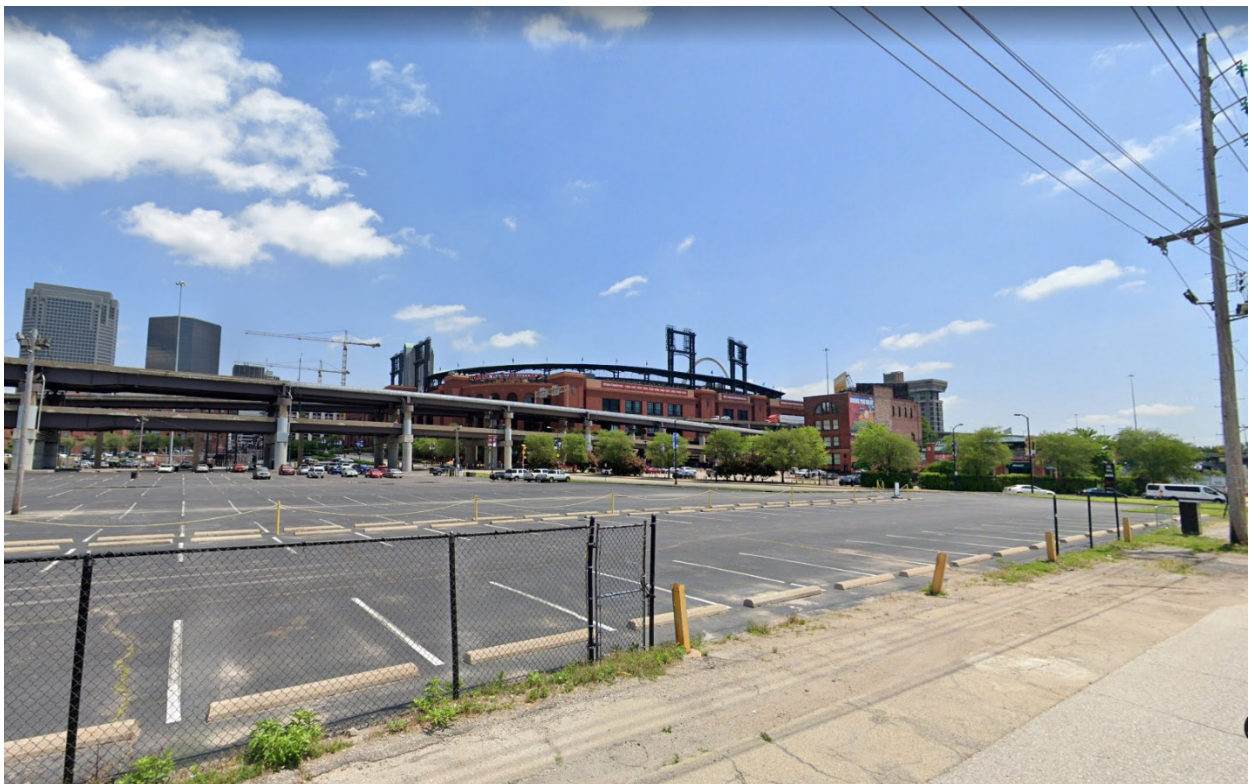
Existing site conditions - Damaged and missing fence along Cerre
