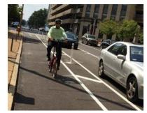
The new parking-protected bike lane stretches along Chestnut Street between 4th and 20th Streets using parked cars and flexible posts to separate the space for people to ride bikes and the driving lane. A striped buffer painted on the street also creates space between open car doors and the bike lane where people are riding.
