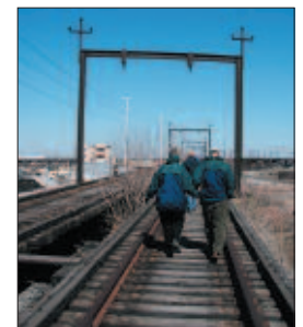
McKinley Bridge and Branch Street Railroad Trestle
